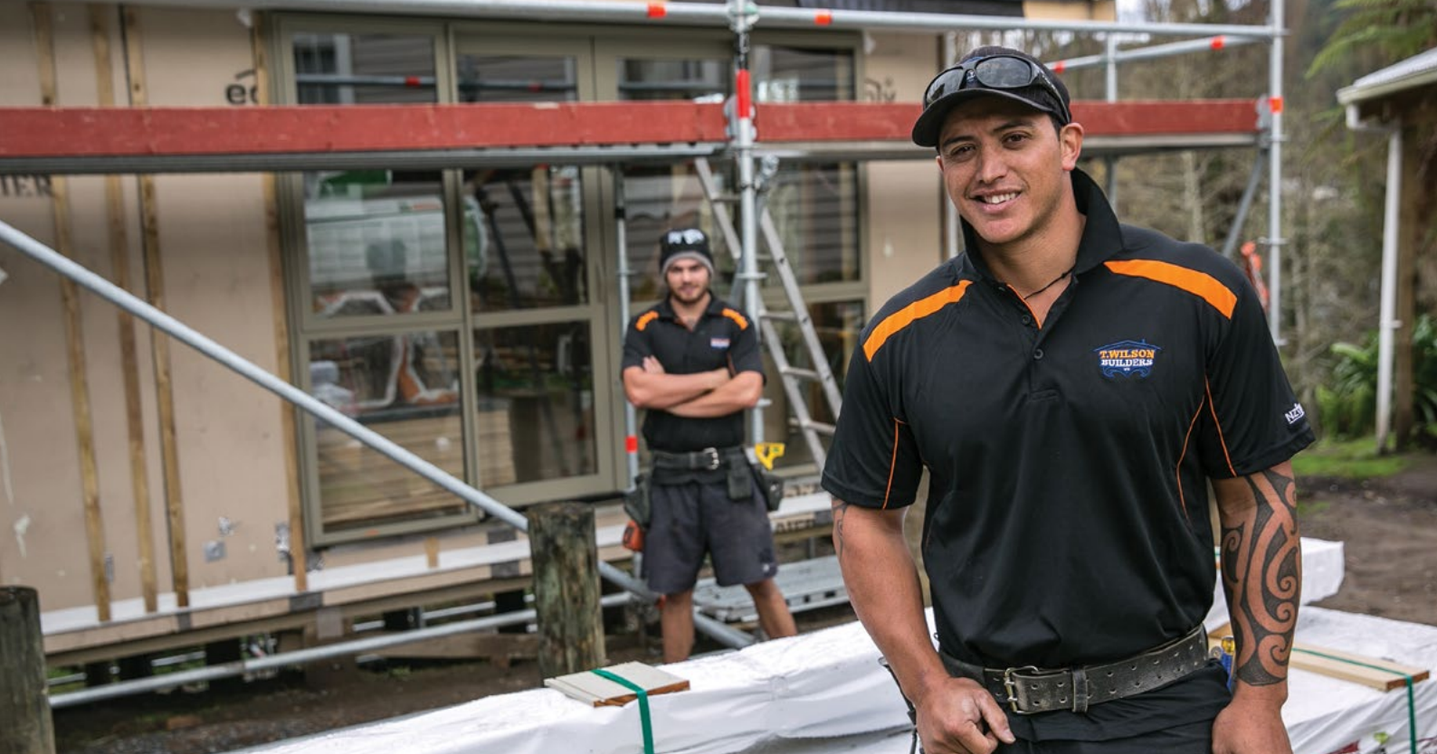
Tyler Wilson and one of his builders on site in Hamilton. Tyler owns T.Wilson Builders based in the Waikato. Photo credit: Rāwhitiroa Photography.
